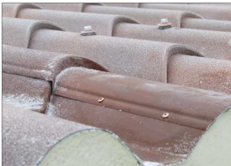
Example of correct rivet use
